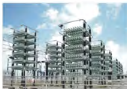
TBB525-301824/S24ACW 并联补偿电容器在±800KV特高压换流站运行 TBB525-301824/S24ACW Shunt Capacitor Installation for ±800KV Ultra-high Voltage Converter Substation in Guangdong Province
