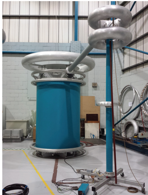
500 kV power transformer with PD testing
