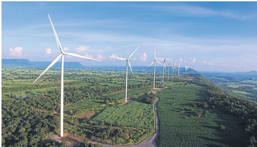
Gunkul Engineering's wind farm in Nakhon Ratchasima's Sikhiu district.
